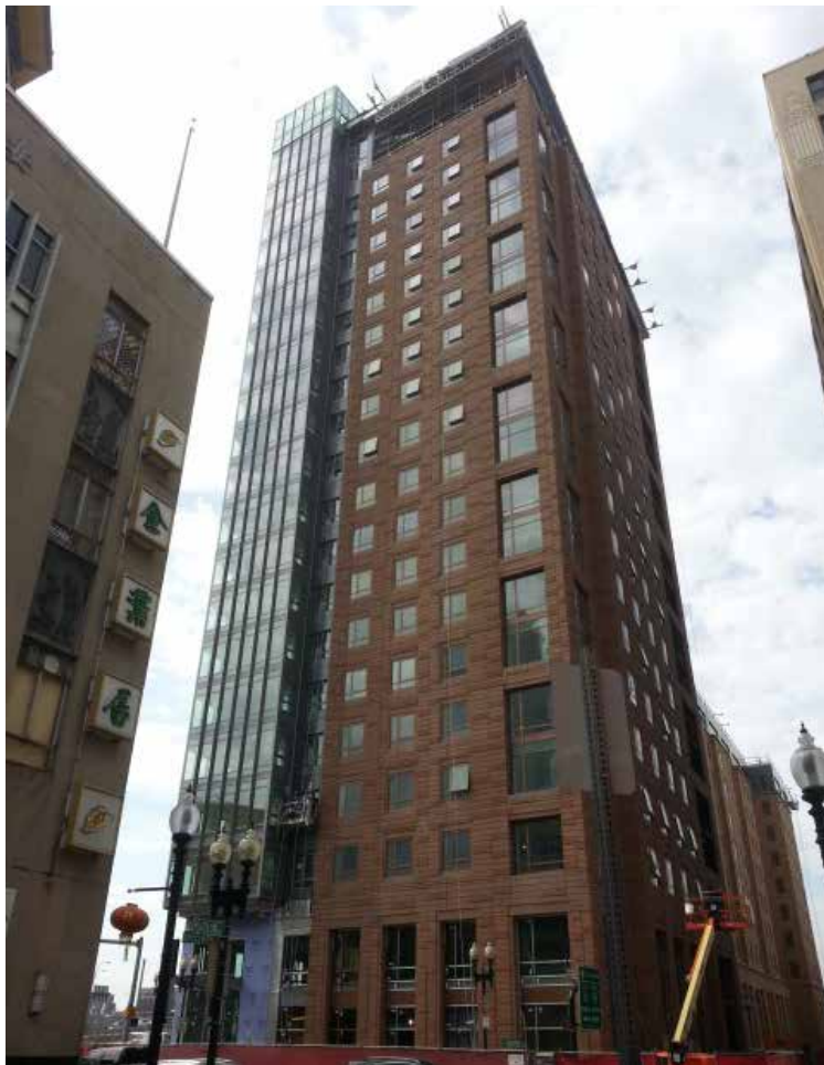
The Urban Strategy America Fund partnered with the Asian Community Development Corporation to develop One Greenway, a major mixed-income development in Boston's Chinatown neighborhood. Two residential towers bookend an acre of publicly accessible open space and a new pedestrian connection. The 312-unit North Building comprises 217 market-rate and 95 affordable rental units.
