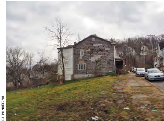
Vacant land and houses that are in disrepair like this one in Esplen are located throughout the study area and surrounding areas.
