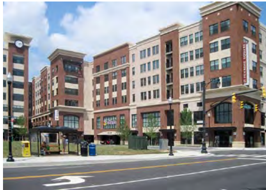
Penrose Square on Columbia Pike in Arlington County, Virginia, was formerly the Adams Square Shopping Center. The project includes 299 residential apartments, a 61,500-square-foot grocery store, 36,000 square feet of additional retail space, and 713 parking spaces. Arlington County paid for 122 parking spaces to be reserved for public parking. A redevelopment like this project should be a longer-term goal, potentially for when leases begin to expire at the Shoppes at Chartiers Crossing and demand for new rental construction increases.
