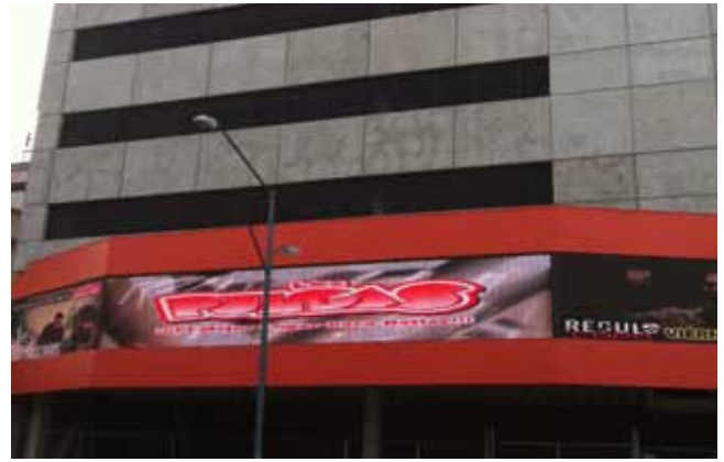
Parking Structure Adjacent to Las Pulgas
