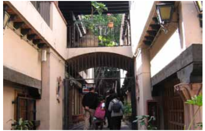
Existing space between buildings in the Demonstration Block
