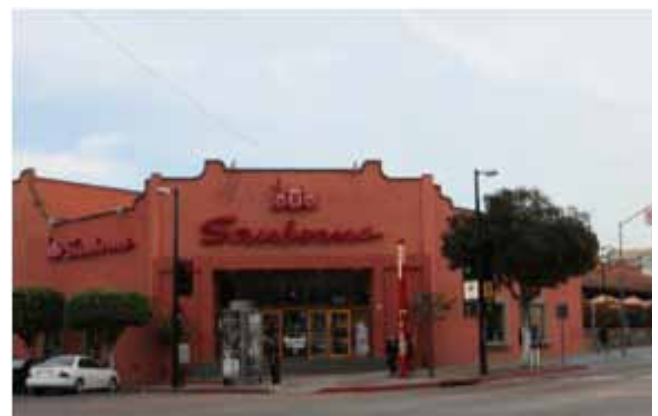
The Sanborns Building
