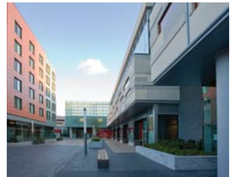
The L-shaped plaza in Harper Court, as seen from the 53rd Street entrance, with the hotel on the left. This street/plaza is owned by the developer and can be closed for community events.
