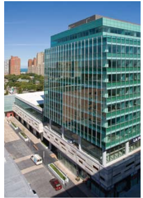
The office building rises 12 stories, providing views of Lake Michigan, the University of Chicago, and downtown Chicago. The office space is 100 percent leased to the university.
