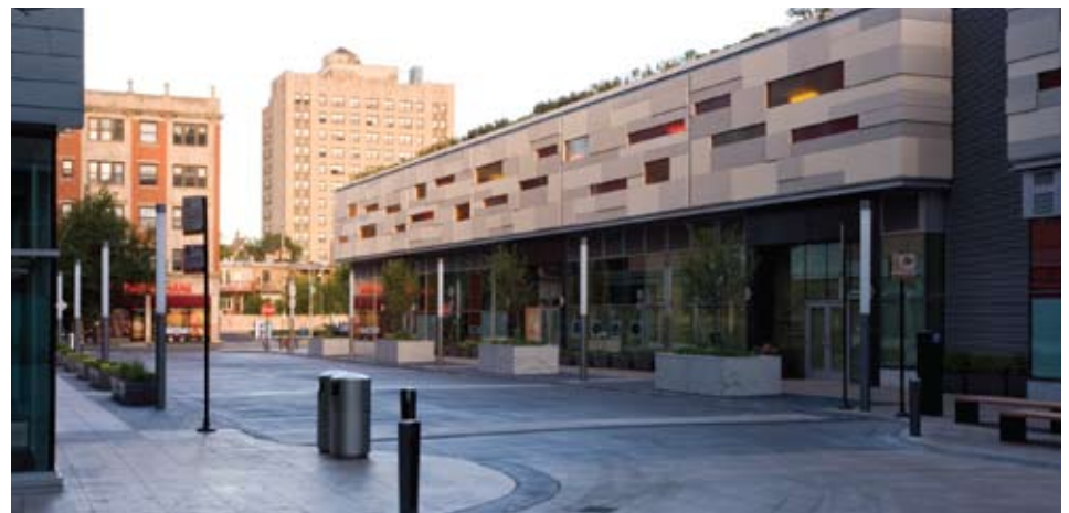
The internal street in Harper Court as it turns toward South Harper Avenue. Storefronts in this area are devoted to restaurants and other food services. Structured parking is on the second level, with open-air parking on the third level.
