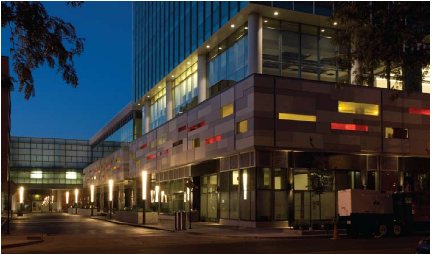
The parking-level windows add color and light to the space at night, unlike most parking garages, which often have harsh white lighting. Pictured is the office building as seen from 53rd Street.
