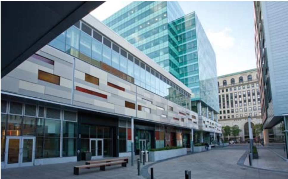
The office building and the internal street as seen from the court looking toward 53rd Street. On the ground level are retail space and lobby entrances. The second level includes parking hidden behind a beige facade with colored windows. On the third level is the LA Fitness health club.
