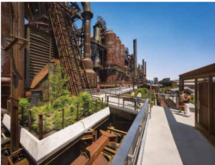
The Hoover-Mason Trestle is a new structure that was placed above and in some places next to the existing rail trestle; the original trestle was used to deliver materials to the blast furnaces.
