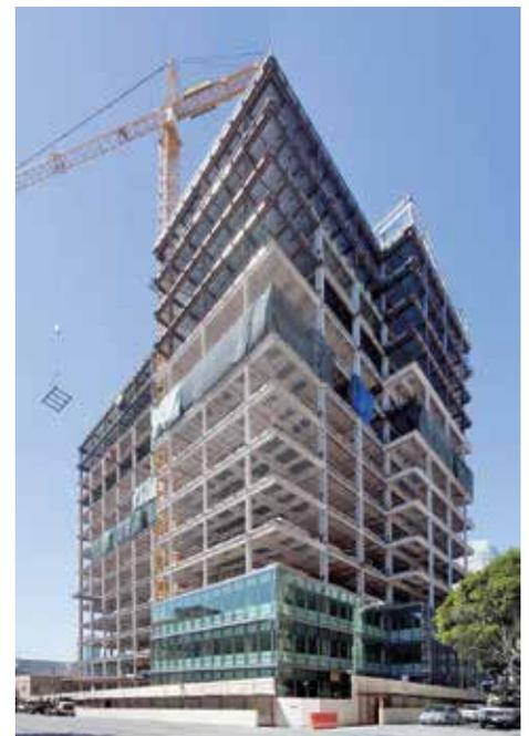
*The building facade was removed and replaced with high-performance glass.*
