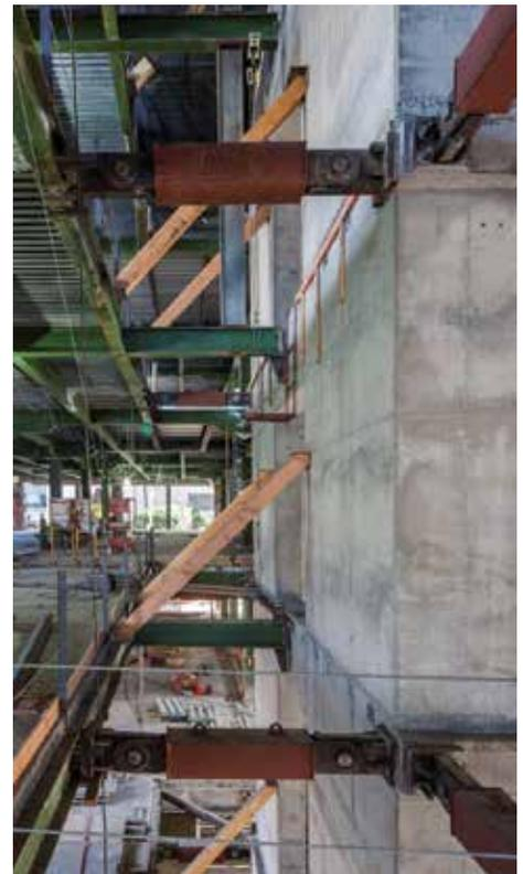
*Horizontal braces link the new concrete core of 680 Folsom to the existing steel frame. The building has been seismically retrofitted to exceed building code requirements.*
