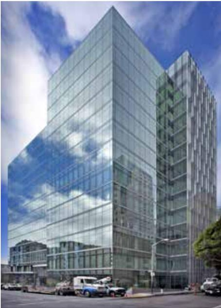
*The 680 Folsom building was expanded both vertically, with the addition of two floors, and horizontally, including an extension to both the front and side of the building, highlighted in this image.*
