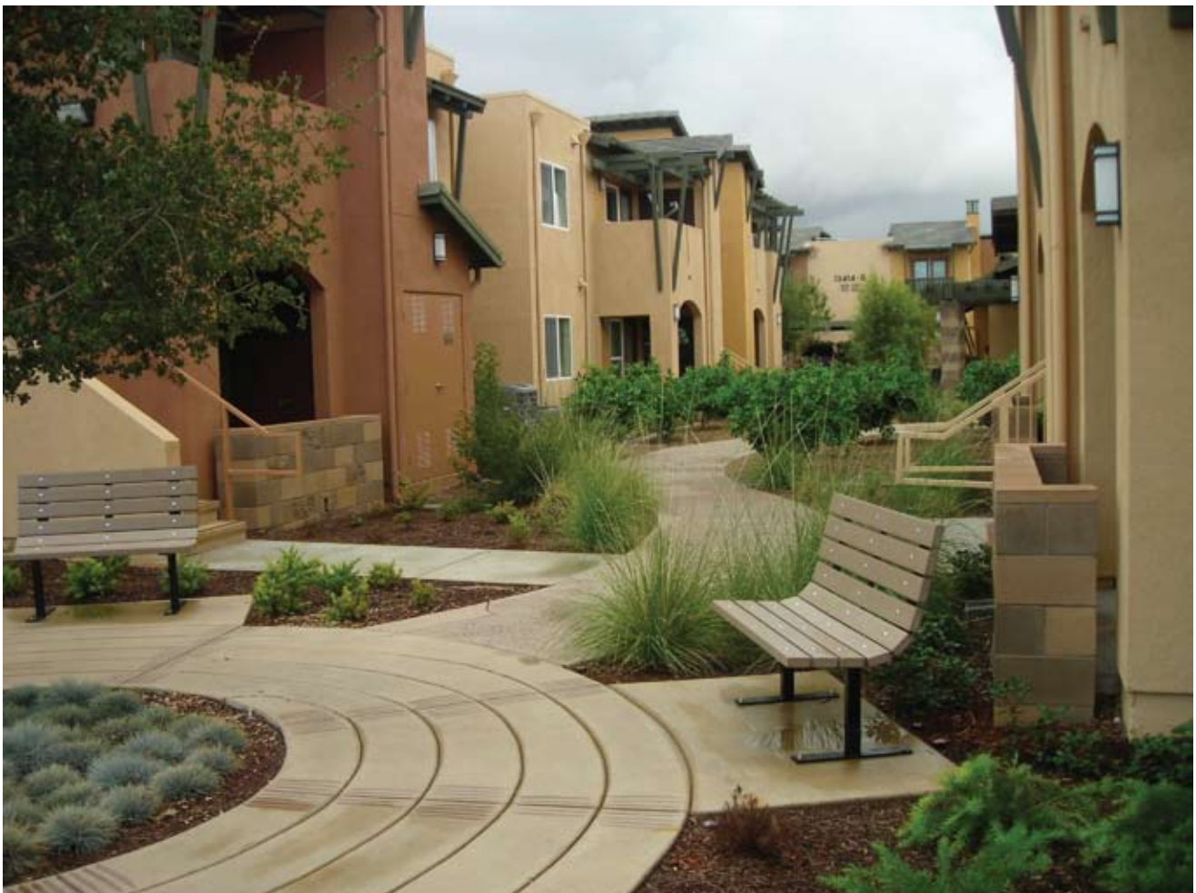
Solara is the first fully solar-powered apartment community in California.
