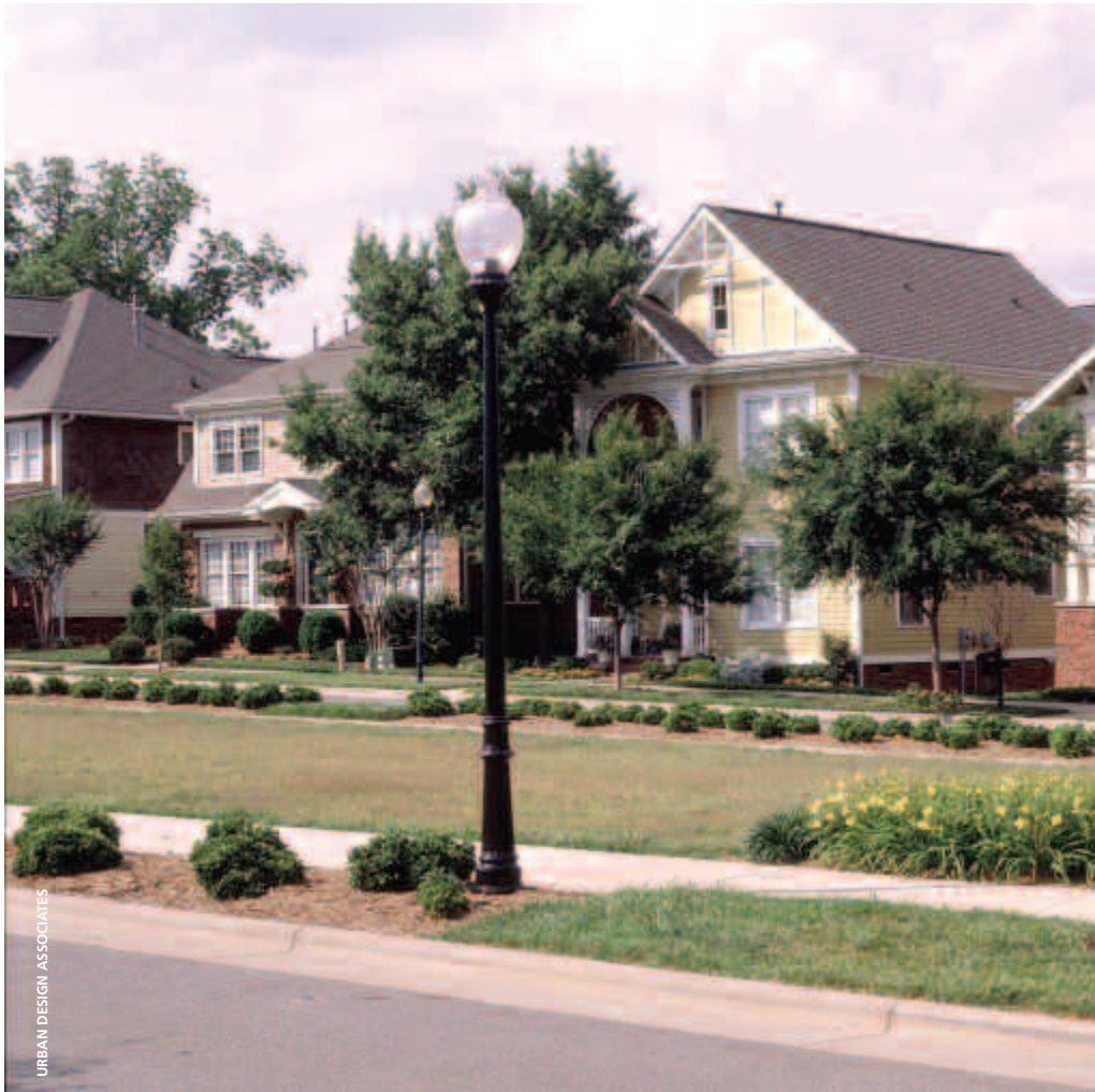
To create a sense of community, traditional town planning principles associated with new urbanism were employed at First Ward Place in Charlotte, North Carolina. The site was developed by the Bank of America Community Development Corporation and the Charlotte Housing Authority.
