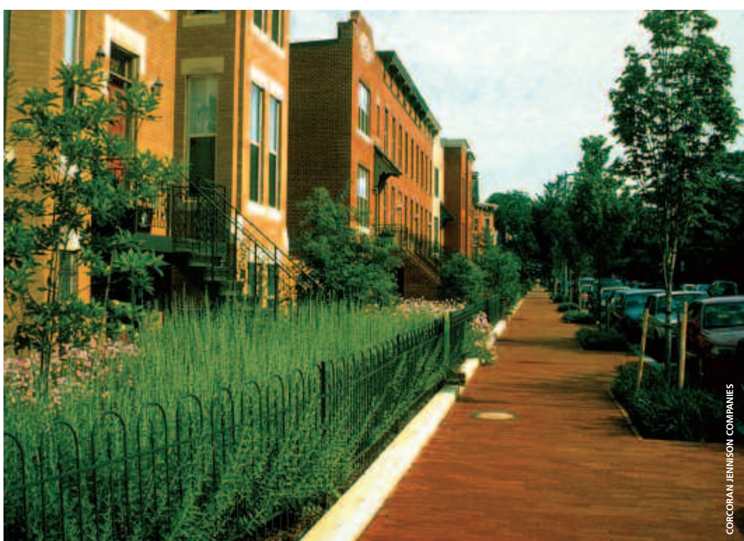
The Townhomes on Capitol Hill in Washington, D.C.—a project financed through a HOPE VI grant—blends seamlessly into the existing neighborhood. Corcoran Jennison Companies, a Boston-based for-profit developer, served as development and marketing adviser and general contractor, and is property manager.
